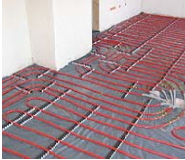
Underfloor heating pipes, before they are covered by the screed
