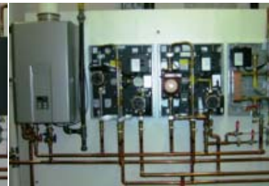
Modern factory assembled hydronic control appliances for underfloor heating and cooling, shown with covers off.
