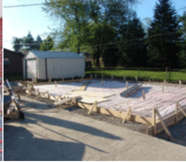
Underfloor heating pipes, before they are covered by a concrete garage slab
