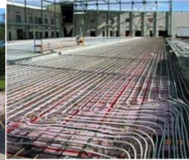
Radiant tubing layout, Project: BCIT Aerospace Hangar, Vancouver, British Columbia, Canada
